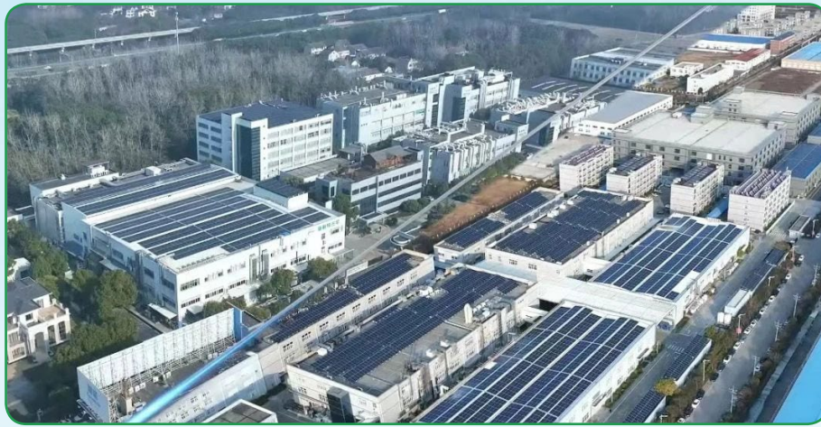
The Group's Production Bases Incorporating Distributed Photovoltaic Power Generation Systems
